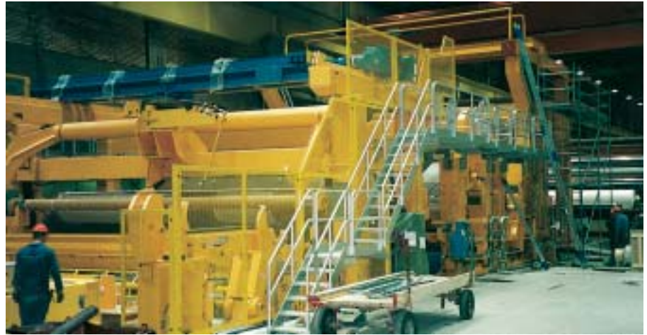
Fig. 3: To shorten erection time a completely preassembled hood portion at the coating section was mounted as a whole.
