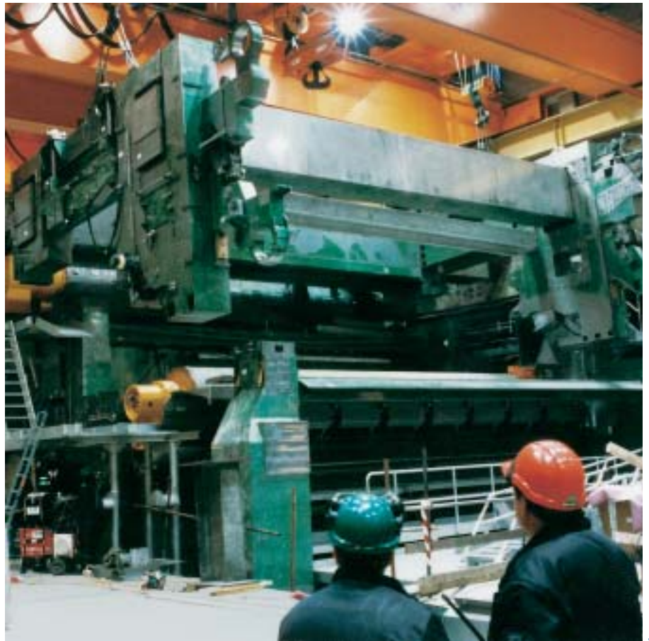
Fig. 5: The framing of the wet end was preassembled before being mounted by crane.
