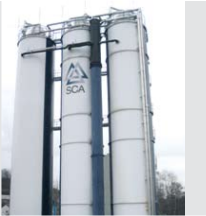
The converted reactor at SCA Aschaffenburg, Germany (center).
