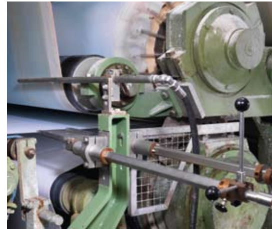
Improving operator safety by installing a TailDeflector for tail threading in the press section.
