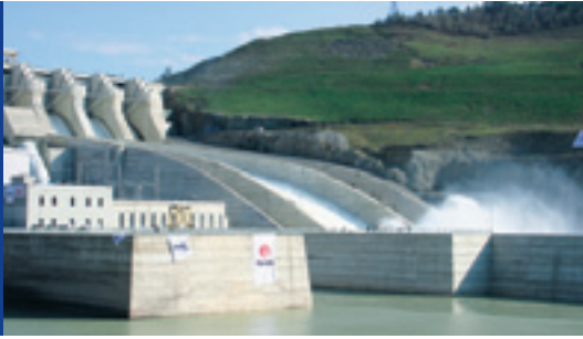
Hydro Power Plant Borçka at Çoruh river in the north of Turkey
