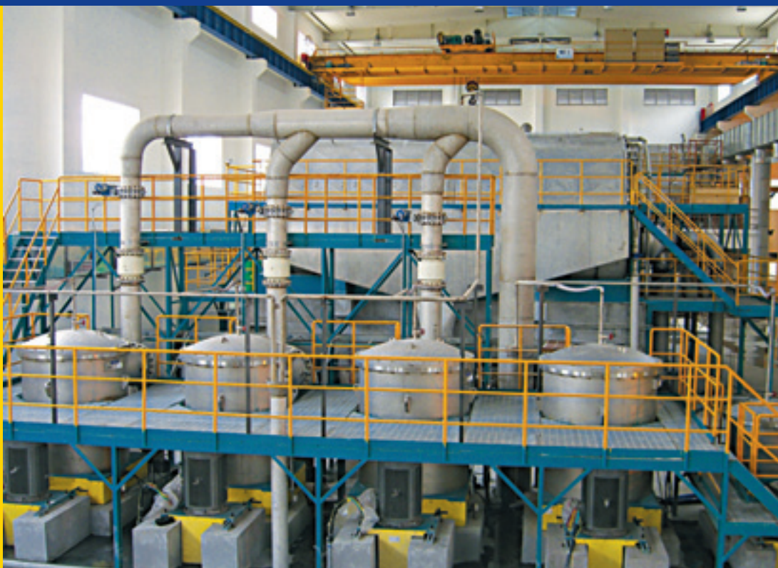
MultiScreen MSS fine-screen system.
