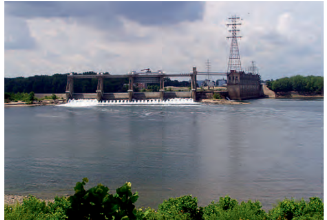
The Ohio Falls Hydro Station is gaining a significant capacity boost.
