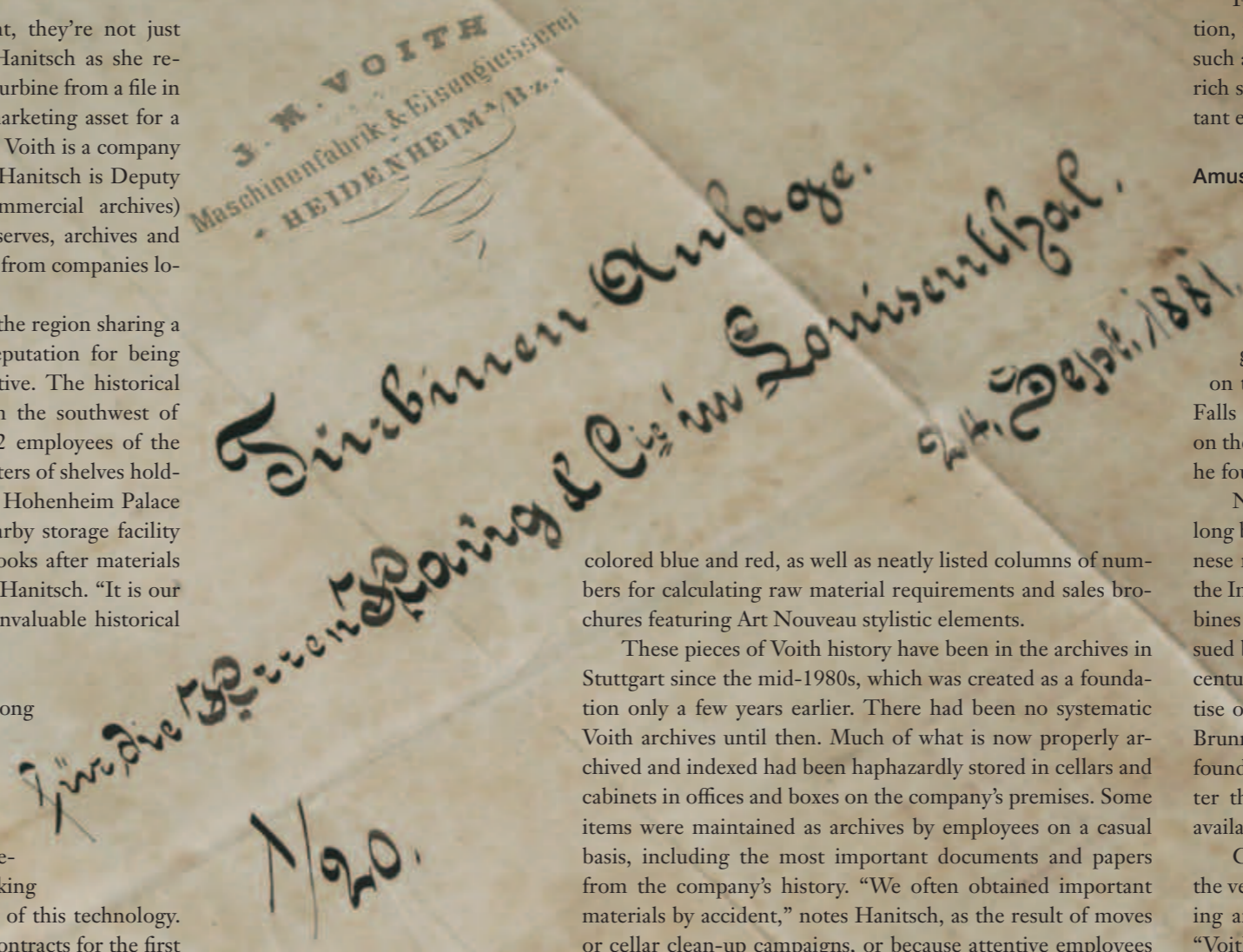
Witness to a long history: a turbine construction drawing from 1881 for a customer in Bavaria.
