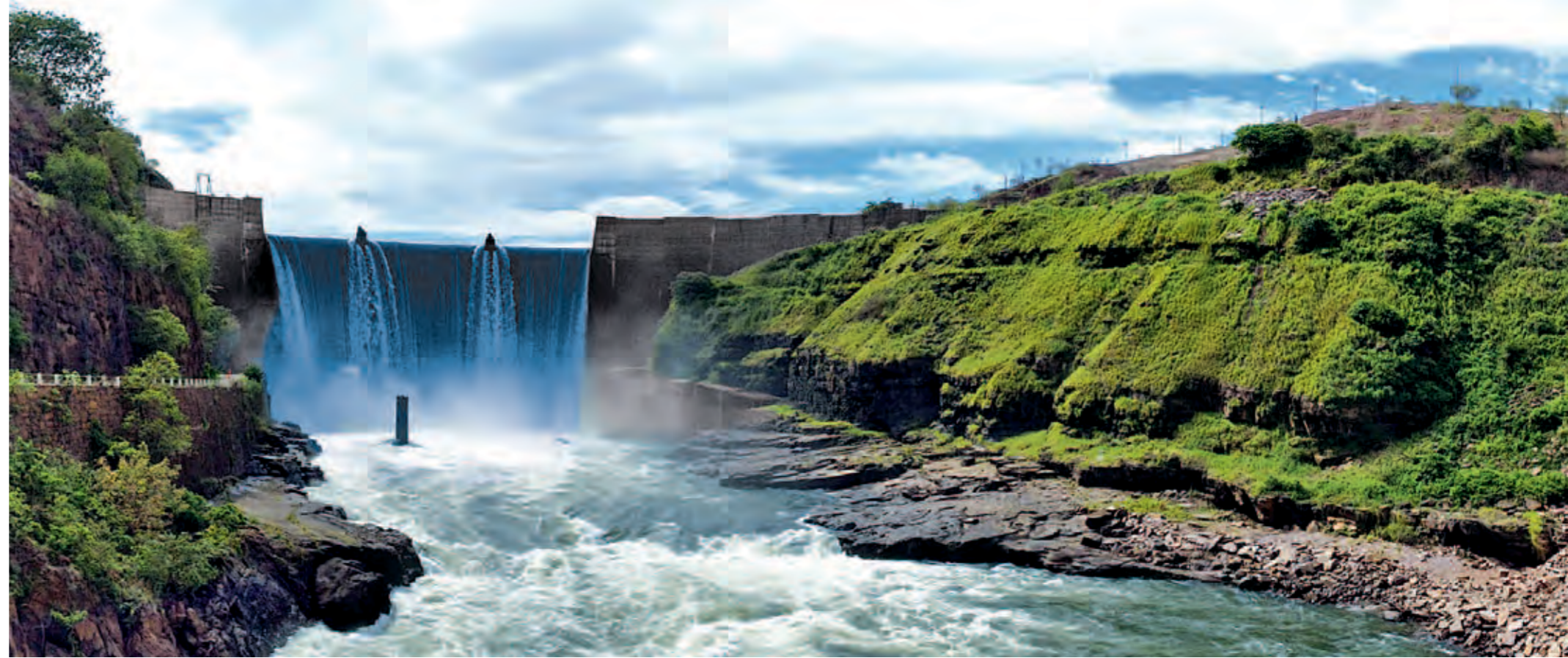
Voith has completed a major upgrade of the Cambambe plant on the Kwanza River. Now, a second plant is planned for the region.
