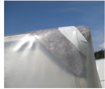
Figure: Lining sharp edges
